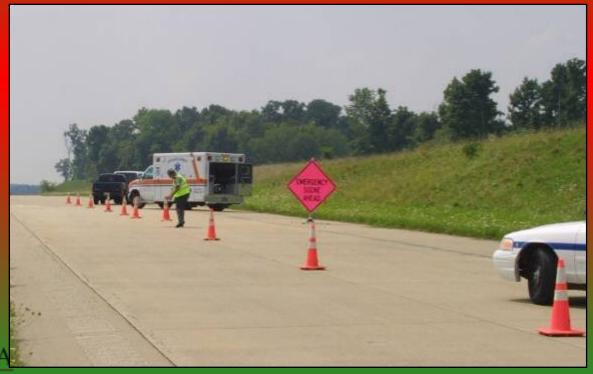
10. Assign personnel to monitor approaching traffic and activate an emergency signal if the actions of a motorist do not conform to established traffic control measures in place at the highway scene.
