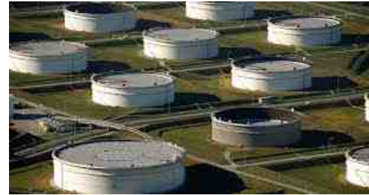
Floating Roof Tank
