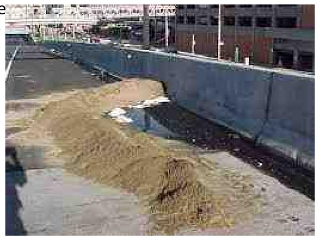
Retention-Building a dike to encircle the spilled product, holding it in place.
